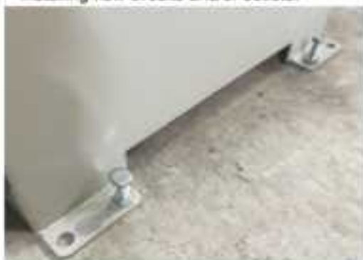
Figure 7-1 Leveling Bolts and Nuts
